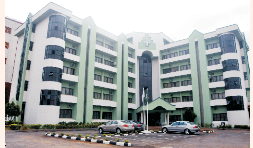
NHRC Headquarters, Abuja
